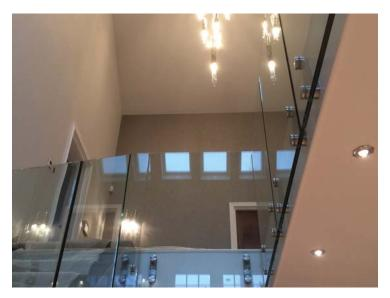
Glass balustrades are designed to provide edge protection to stairs, landings, lightwells, ramps and any other circumstance where there is the possibility of a fall. Modern glass balustrades minimise the visual weight of the balustrade which could otherwise detract from the aesthetics of the internal finishes or external view. We can supply a multitude of designs from traditional posted systems with infill glass panels to fully bespoke, contemporary styled, point fixed systems.
