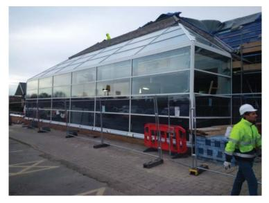
Glazed facades provide any structure with a lightweight glazed infill that provides access, ventilation and natural daylight into multiple areas of the property whilst providing a modern focal point to the external facade. We can supply single, double or even triple glazed varitations to suit the individual requirements of your project. Facades can incorporate solar control coatings, Brise Soleil, intergrated blinds or even switchable LCD Glass options.
