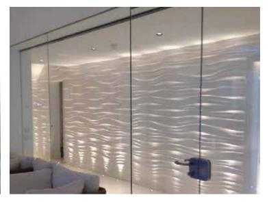
Glass partitions are a quick and easy way to divide large spaces into smaller rooms such as individual offices and meeting rooms, or between different elements such as swimming pools and gymnasiums whilst maintaining the transfer of light between areas and maintaining that open plan feel. Most of our partitions are designed to be frameless where the glass is fitted into recessed channels installed in the surrounding walls, floor and ceiling.
